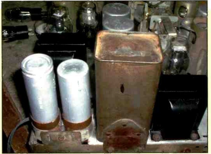
Photo D. The metal cover for the large Philco capacitor bank is back in place, hiding the replacement capacitors from view. Using electrolytic capacitors with high ESR values, instead of Mylar dielectric capacitors, to replace the original wax-paper capacitors caused low-frequency oscillations in the audio stages.
